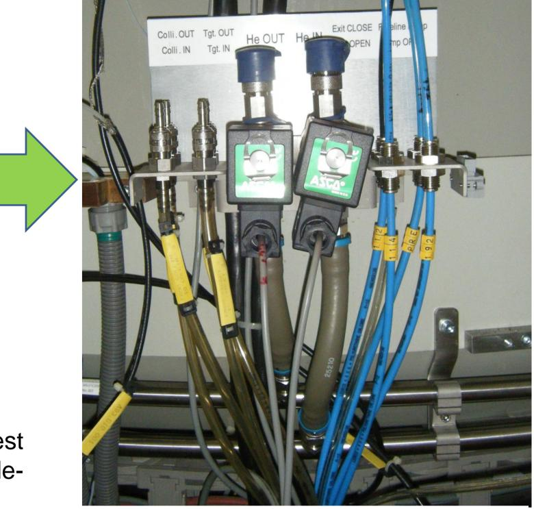
New target manifold; Helium valves & connectors
