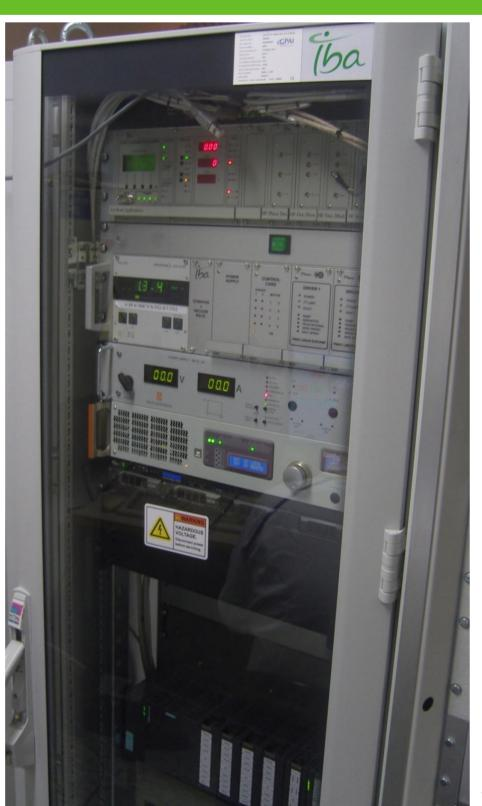
A modern solid state (transistor) pre-driver and a new Low Level RF control unit (LLRF) were installed together in the PLC cabinet (left picture).
